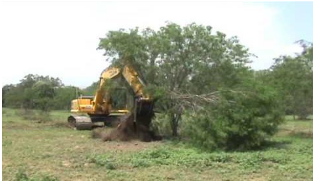
Figure 4: Excavator with Mesquite bucket Attachment 斗式挖掘机
