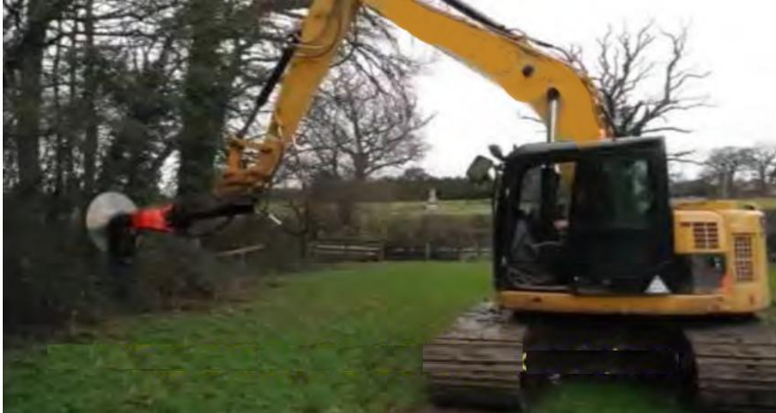
Figure 5: Excavator with Hydraulic Saw attachment 锯式挖掘机
